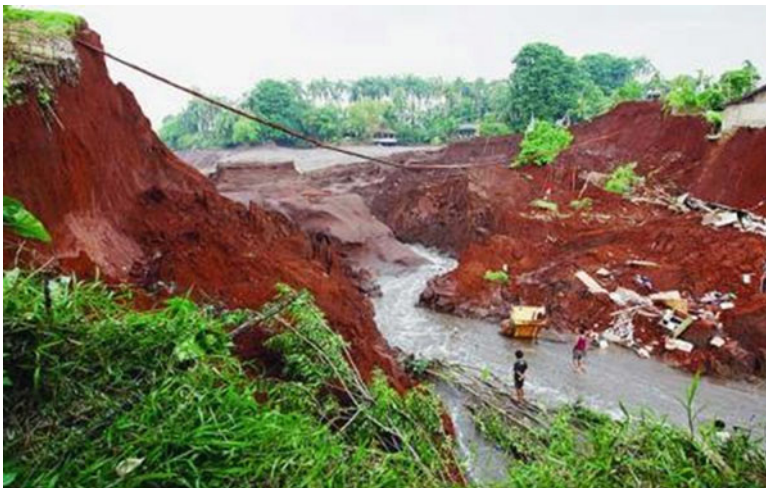
Fig. 4.12 Collapse of the Situ Gintung dam on March 27, 2009
