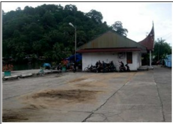
Figure 2 Silty sand liquefaction at Padang airport during 2009 West Sumatera earthquake
